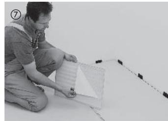
For the third row, peel off the protective film before installing the boards. The film should be removed at a slight angle to prevent it from tearing. Then, starting on the left, the board can be connected and lowered along its long side with plastic dampeners into the already installed rows. Finally, remove protective film from the next board and rotate it downward into place.
