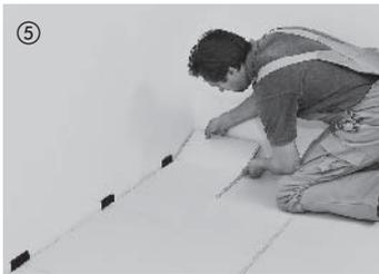
Cut the last board of the first row to size, leaving an expansion gap of 10-15 mm (3/8" - 1/2") between the board and wall. Fit in the board. Start the second row with the leftover piece of the first row (offset the end joints of adjoining rows by at least 18 cm). This considerably reduces waste.
