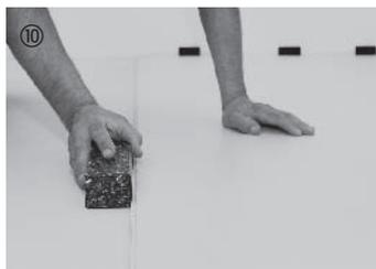
Gently tap along the front edge of the row with the tapping block. Tip: To ensure a strong bond between the boards and the subfloor, we recommend that you walk over each row after installing it. Proceed in this way to install all remaining rows.
