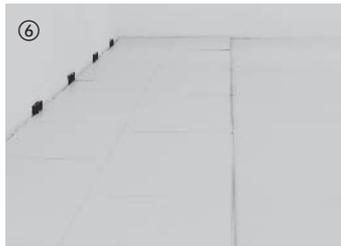
Before laying the remaining rows, it is important to ensure that the first rows are straight and exactly parallel to the wall. When correctly aligned, fix the rows in place with distance spacers. If necessary, the boards can be gently tapped on the long side.
