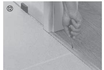
In doorways, mount a suitable moulding system to ensure the necessary expansion space. This also applies if the same floor is to be laid in the adjoining room. Leave an expansion gap of at least 5 mm (approx. 1/4") between the board and the base of the moulding. As a rule, a fine saw must be used to cut a gap the thickness of a board in wooden door frames to allow Celenio to expand.
