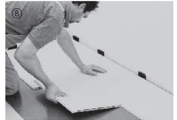
The next row is started with the leftover piece of the first row (short side offset of at least 18 cm). This considerably reduces waste. The rest of the installation is performed board-by-board. First, the boards are angled into the previous row along the long side by applying a small amount of force.
