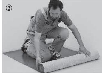
For sound insulation and to smooth out slight irregularities of the subfloor, unroll 2 mm thick luxury insulation layer. Our range of accessories also offers suitable insulation underlays. Asphalt-bitumen felt is not suitable for sound insulation. **Do not use any additional insulation underlay when laying Celenio Silent Pro®.**
